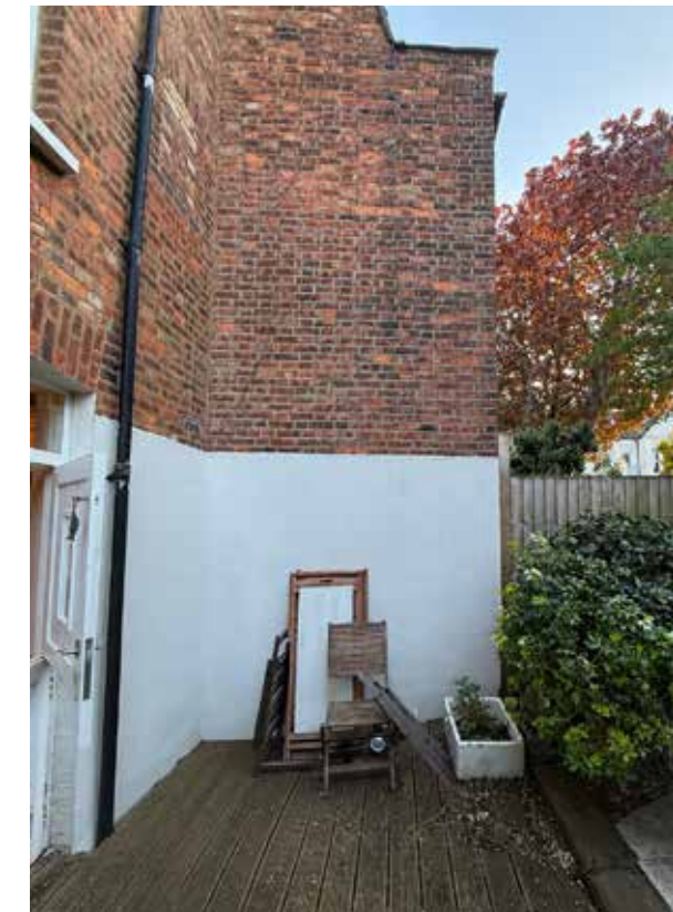
4. Flank wall at No.76-B
