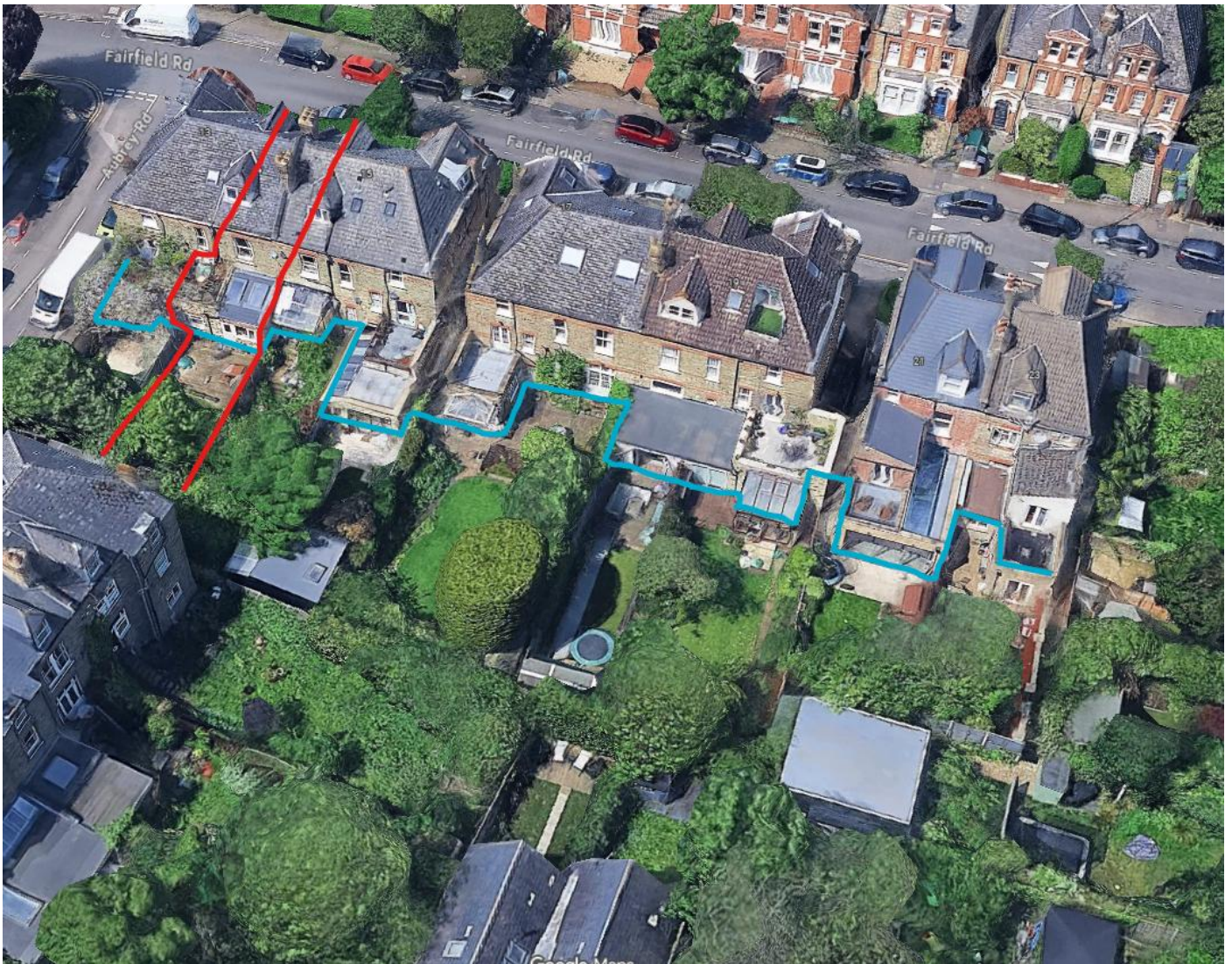
Figure 2 – Building lines to the rear elevations
