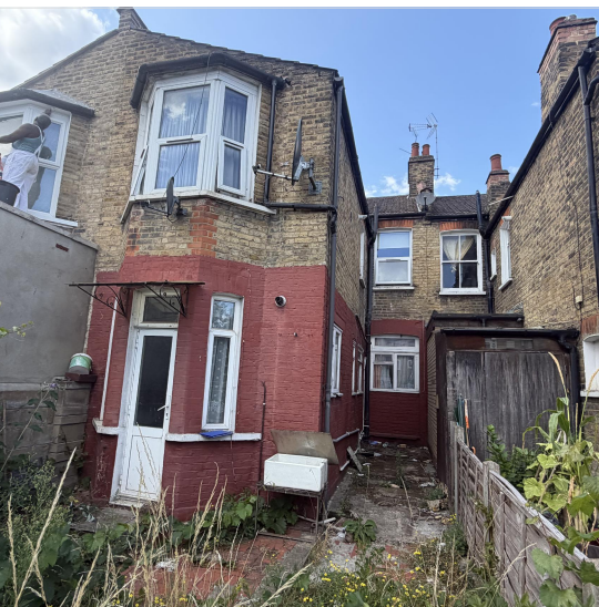
Existing rear view image captured 21st August 2026
