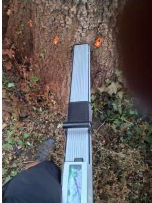
Figure 8: Resistograph drilling in progress in the vicinity of sonic tomography sensor pins 5–9, adjacent to the MP1 test location. (16 August 2026).
