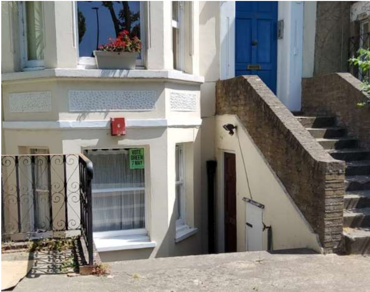
Photograph 2 – adjoining external stair and basement entrance
