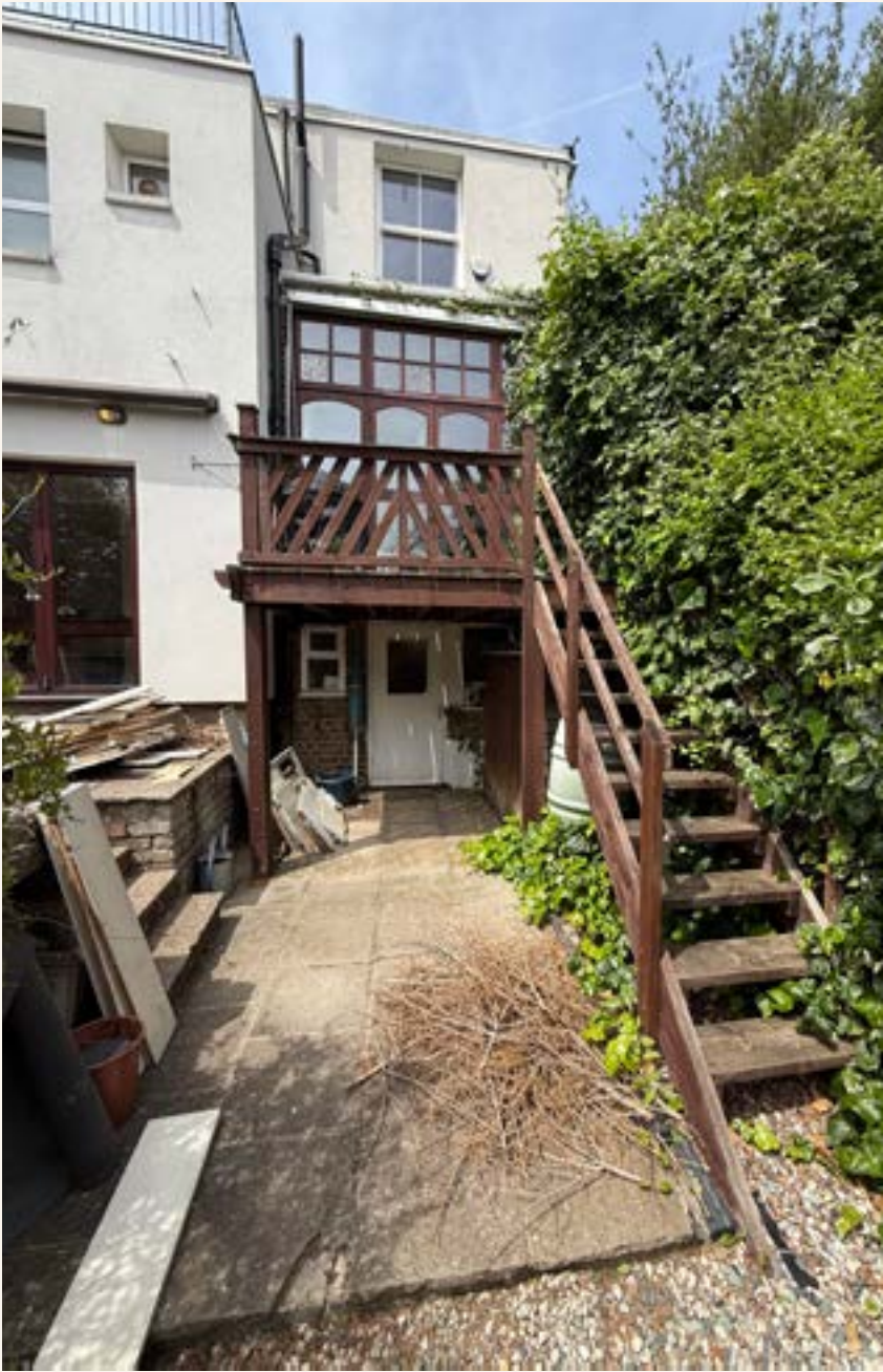
REAR LOOKING TO 63 OAKFIELD ROAD
