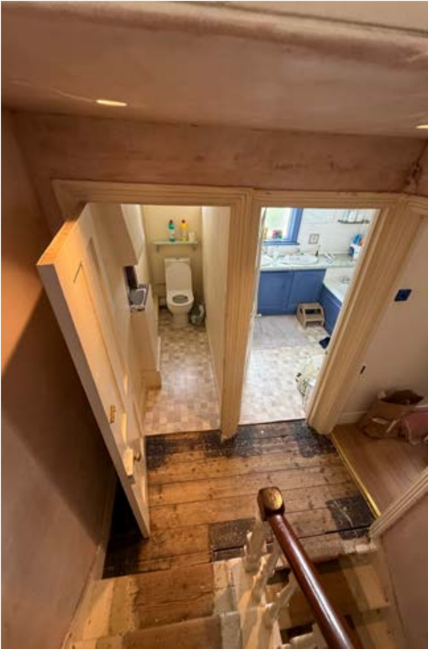
FIRST FLOOR LANDING
