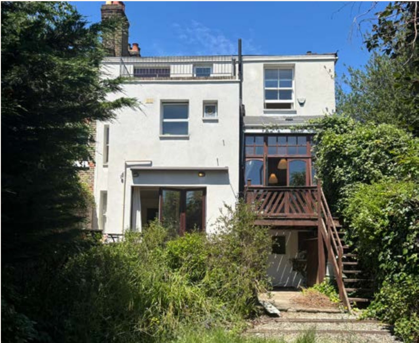
EXISTING REAR ELEVATION PHOTOGRAPH
