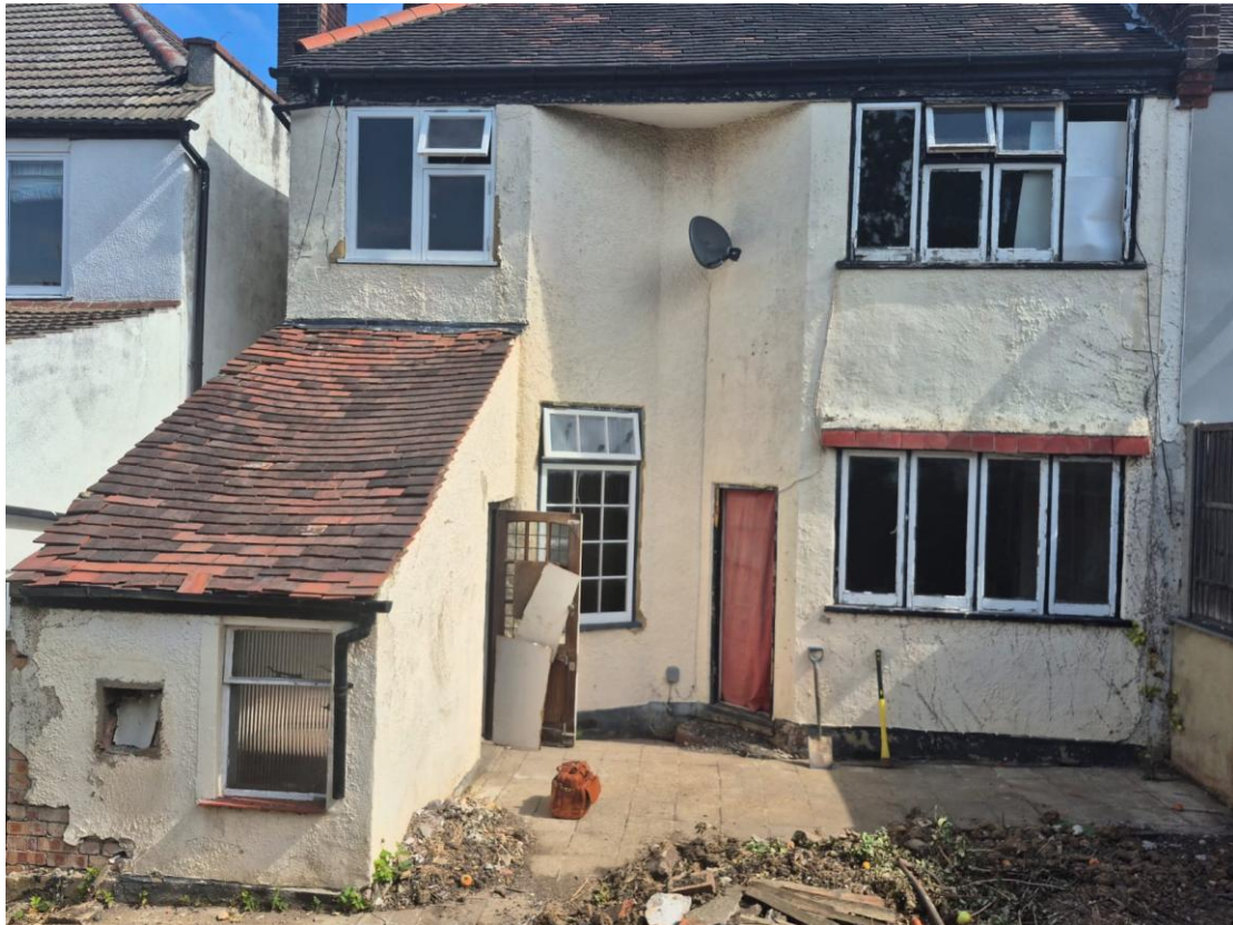
Photo 1 – rear elevation of the existing building.
