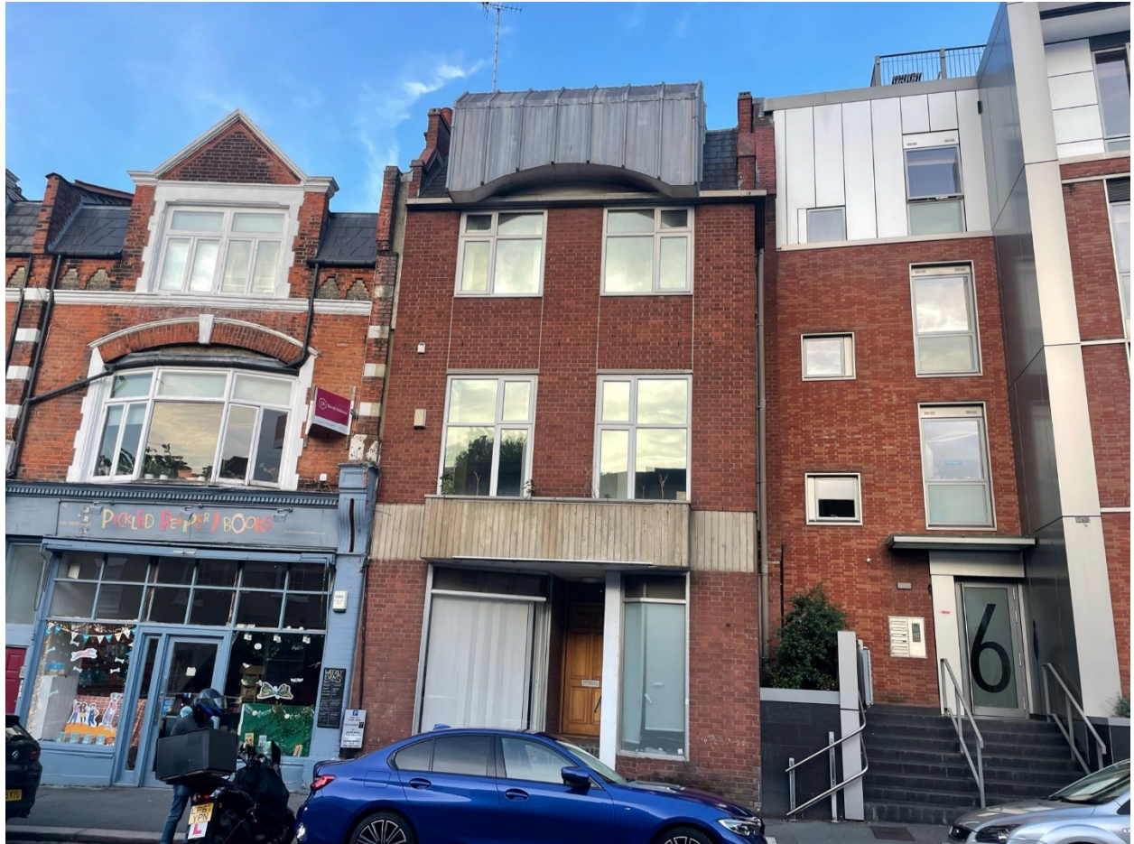
3. Middle Lane – Front View (Greater Context).
