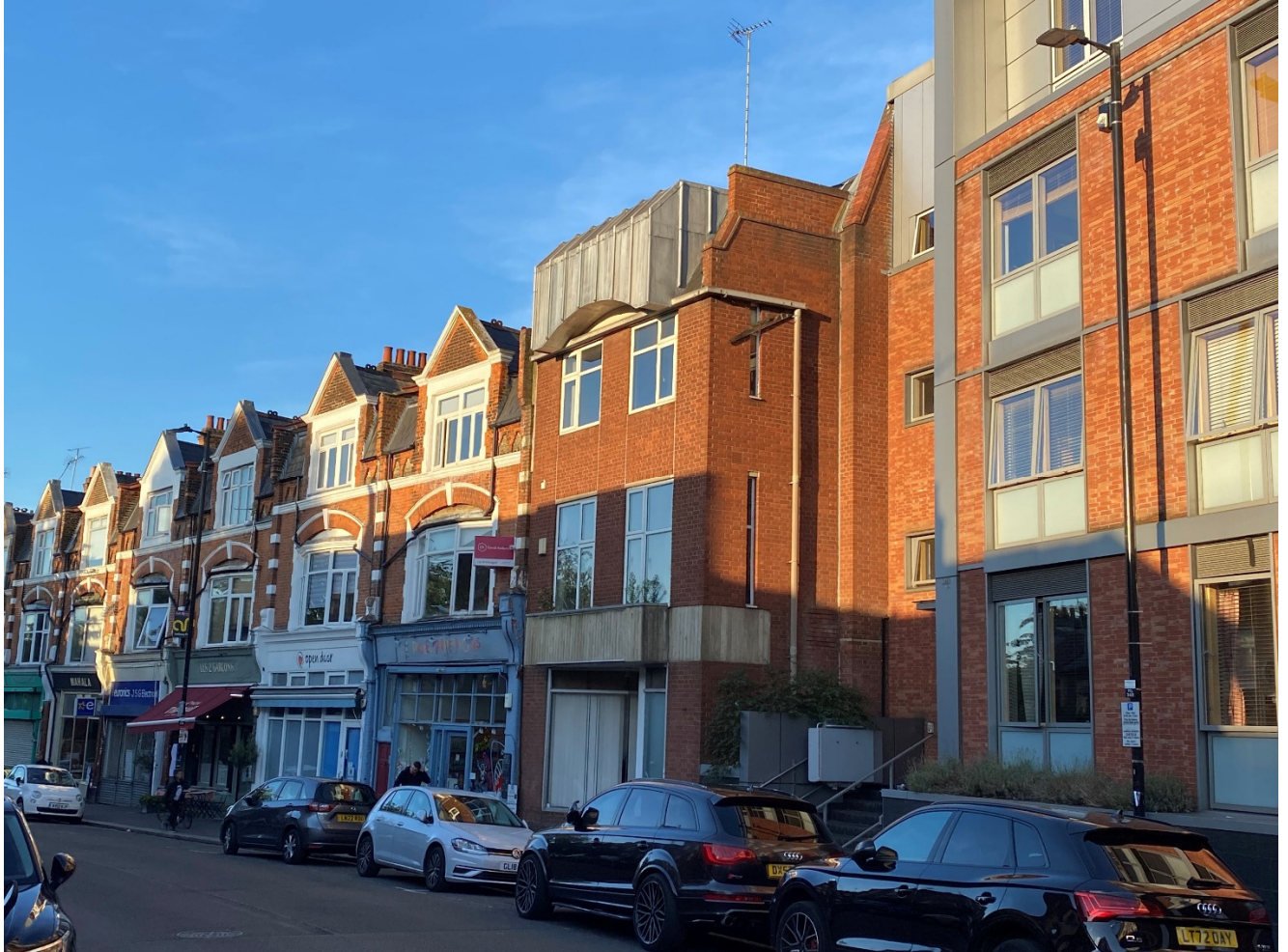
1. Middle Lane – Front/Side View.
