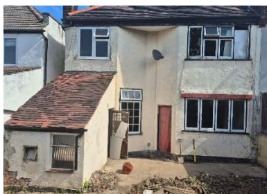
Photo 1 – rear elevation of the existing building
