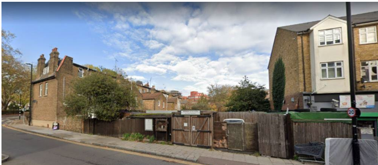
Figure 13 – View of the rear elevation of the application site and adjoining houses on the terrace.
