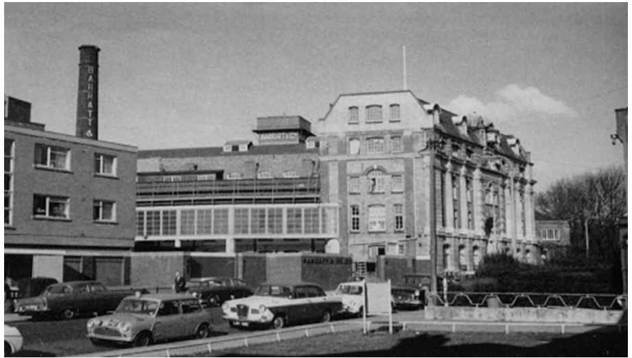
Figure 7 – Photograph of Barrat's office building today known as Cambridge House, a five storey, locally listed office building, erected in 1897 as the headquarters for Barratt & Co Confectioners.
