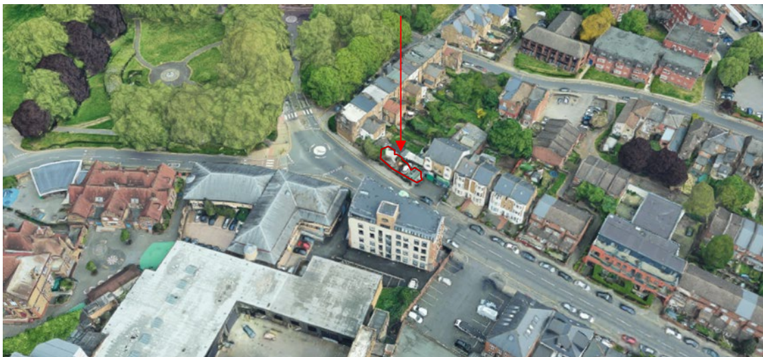
Figure 1 – Aerial View of the site and its context
