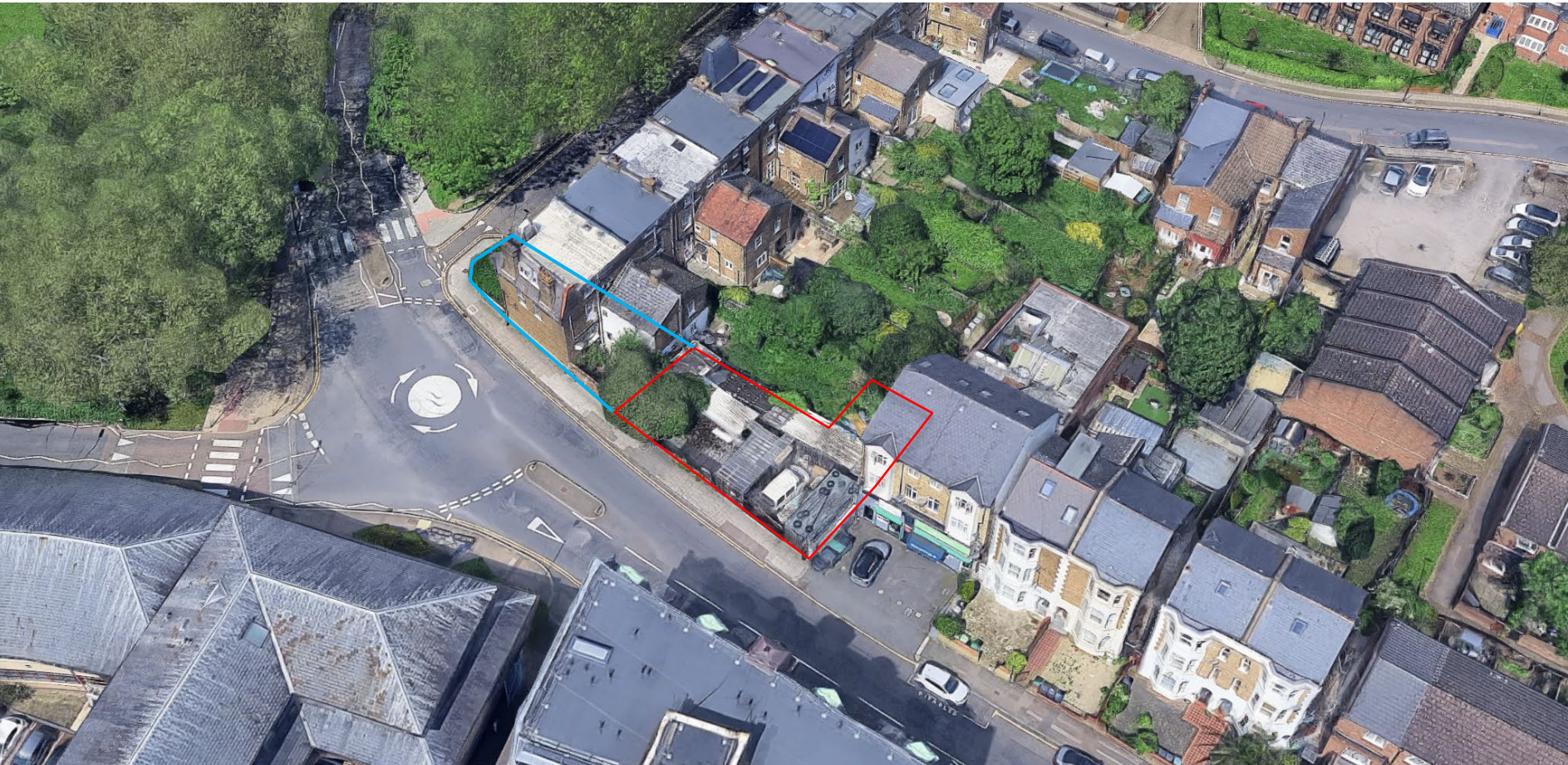
Aerial view - rear
