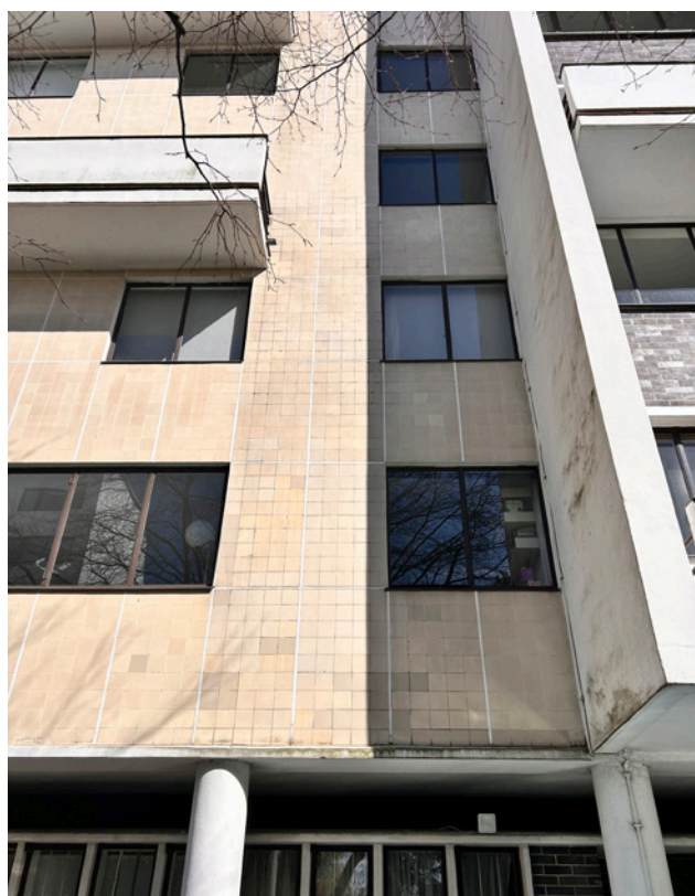
Northern end of rear facade
