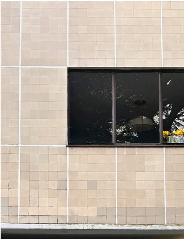
Northern end of front facade - 1st floor
