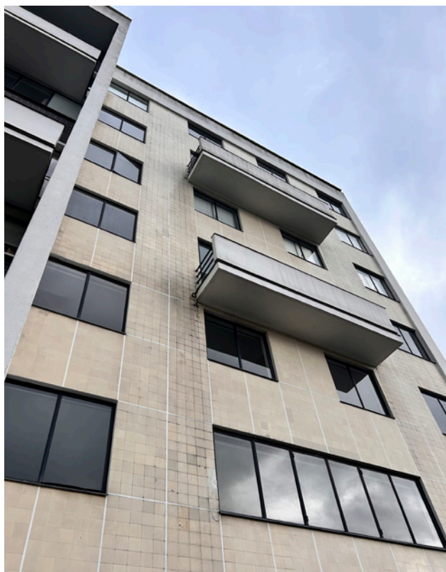
Southern end of rear facade
