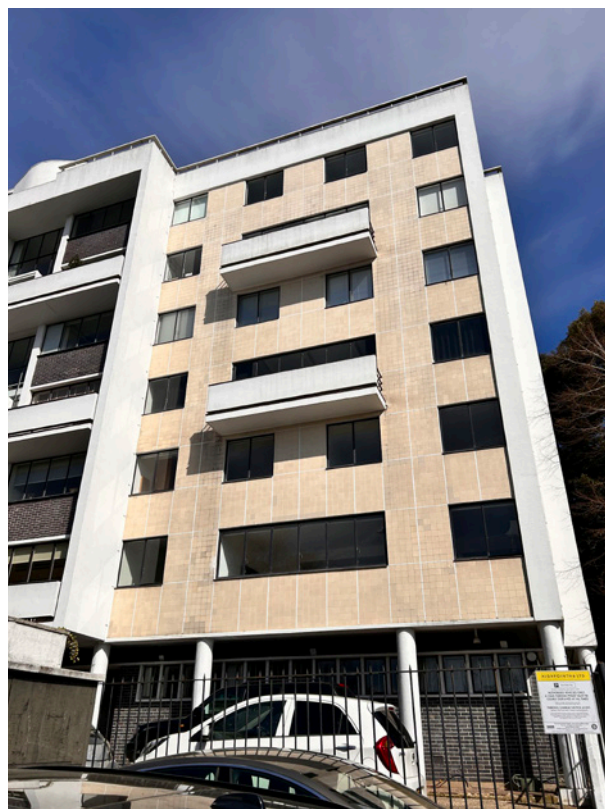
Southern end of rear facade
