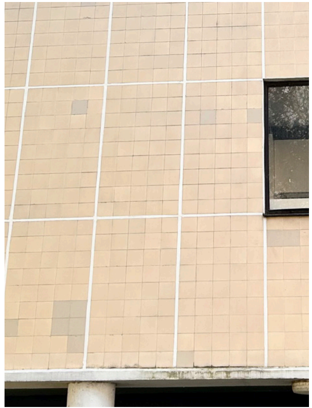
Southern end of front facade - 1st floor
