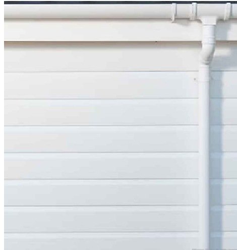
External finish to be white PVC cladding
