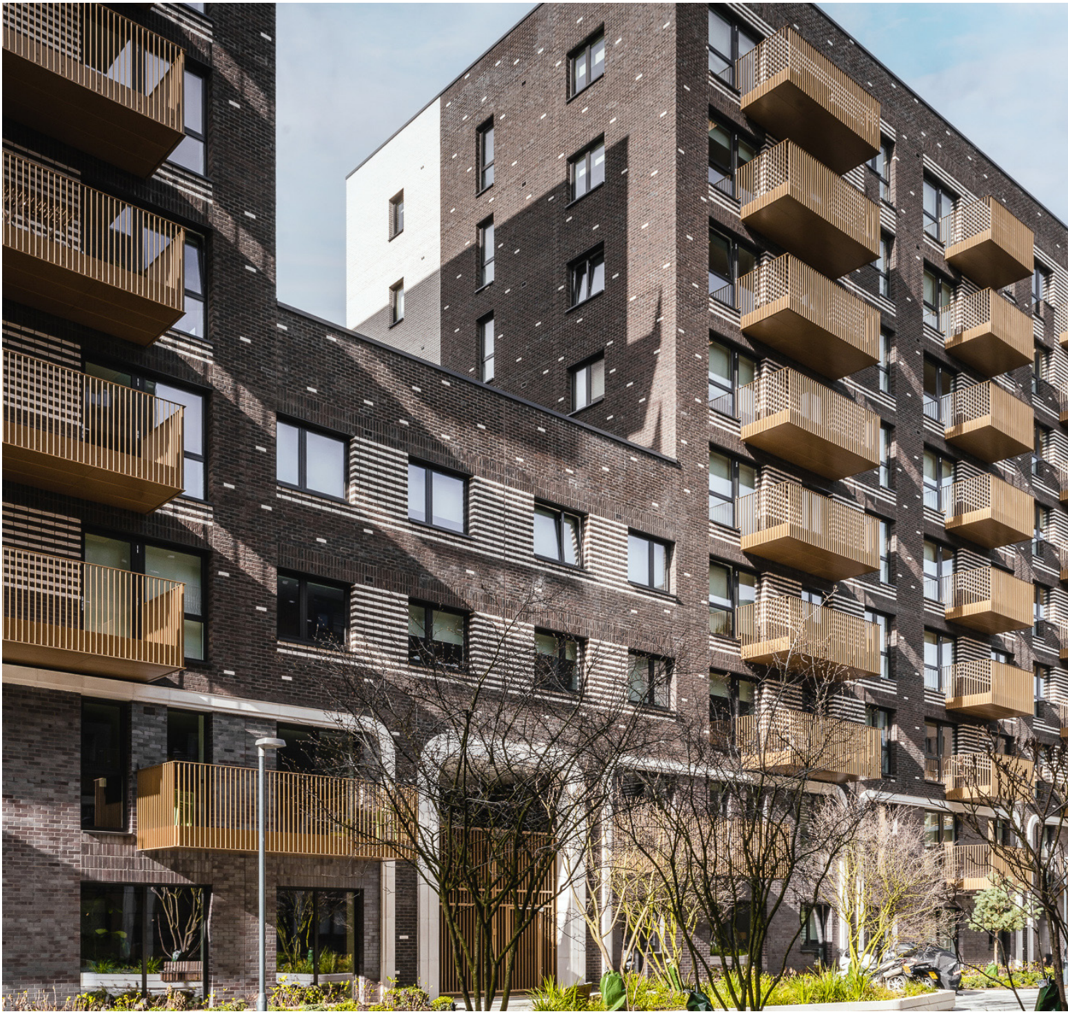
EQUIPMENT WORKS, WALTHAM FOREST
