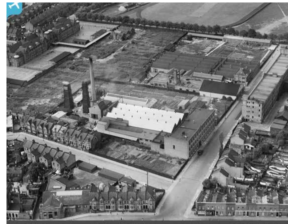
Figure 5.12 Aerial Image of Factories Along Ashley Road, 1933. Source: Britain From Above
