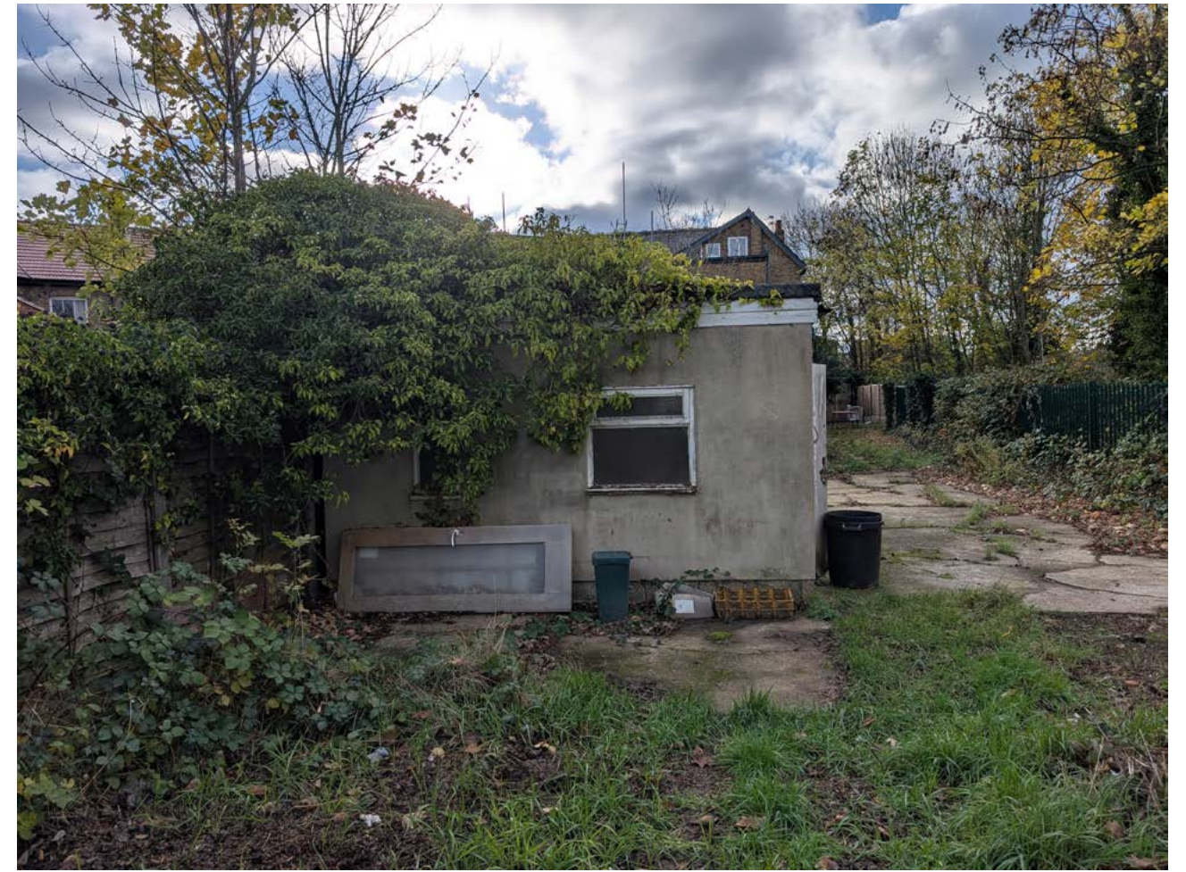
10 - view of garage looking south
