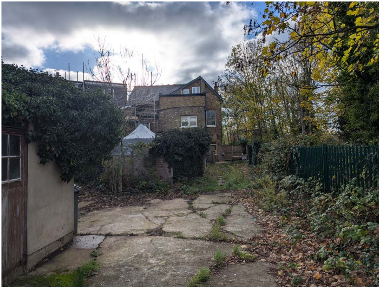
11 - view back to original house from garage
