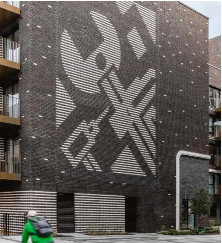
Precedent - Equipment Works
