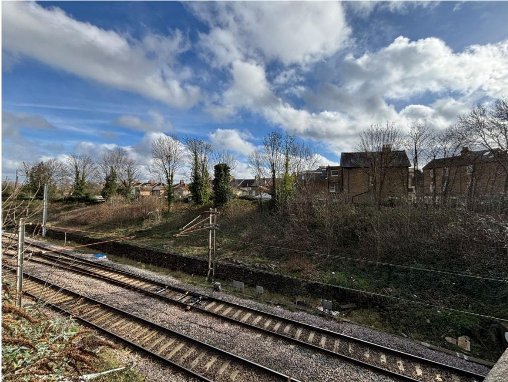
Figure 8: Baseline View 2 looking east from the Bounds Green Road railway bridge.
