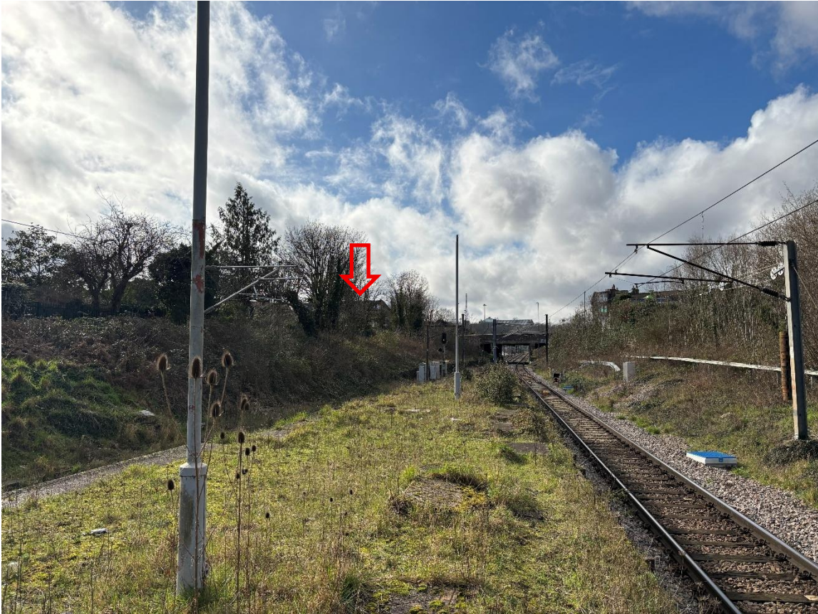
Figure 4: View looking south from Bowes Park Station, the location of the subject site is indicated by the red arrow.
