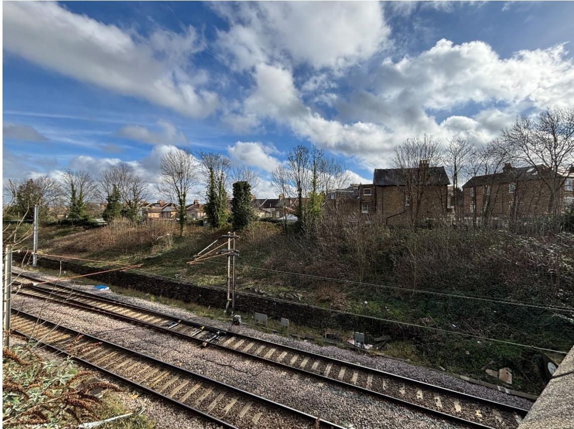
Figure 5: View looking east from Bounds Green Road towards the subject site.
