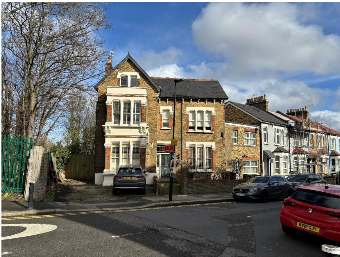
Figure 6: The front elevation of 1 Whittington Road.
