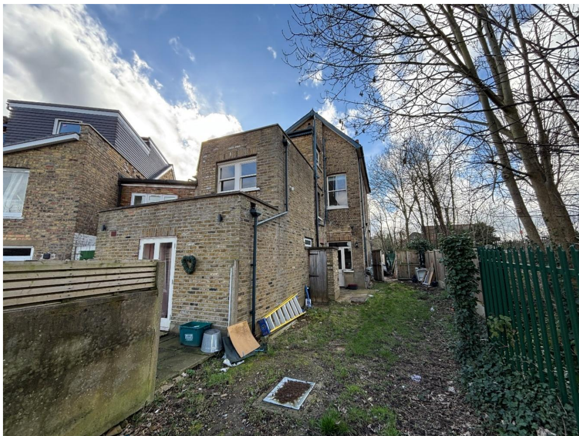
Figure 7: The rear elevation of 1 Whittington Road showing the multiple modern rear extensions.
