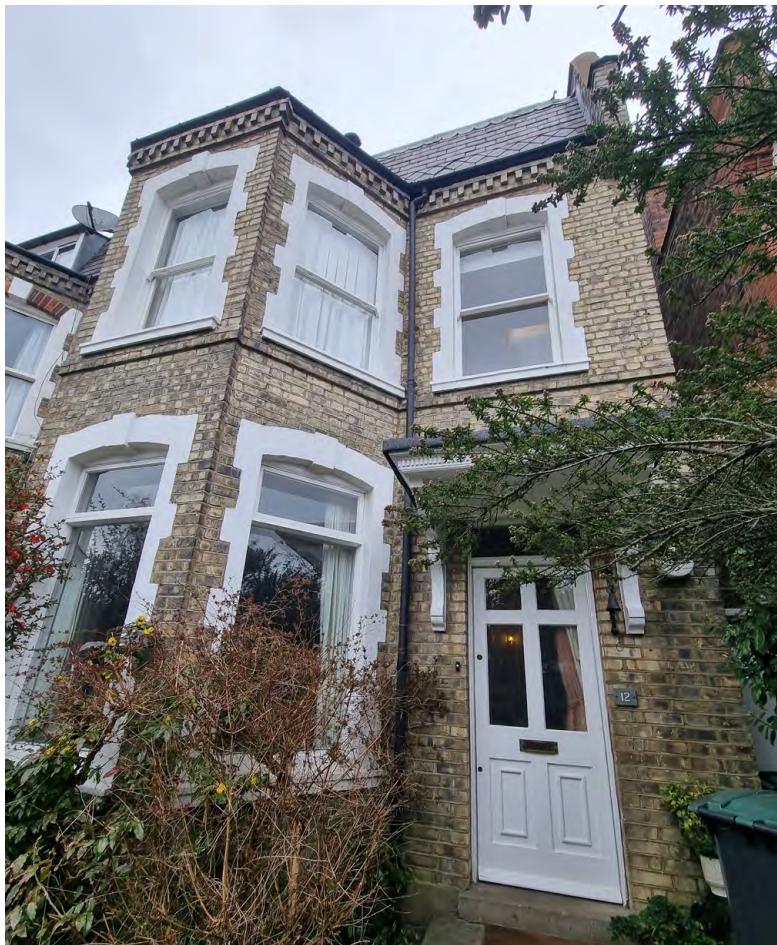
(Fig. 01) Street facing elevation of 12 Southern Road.
