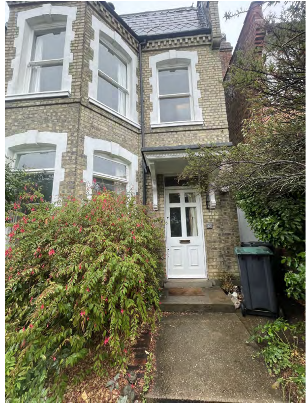
[Fig. 03] Front facade view to 12 Southern Road.
