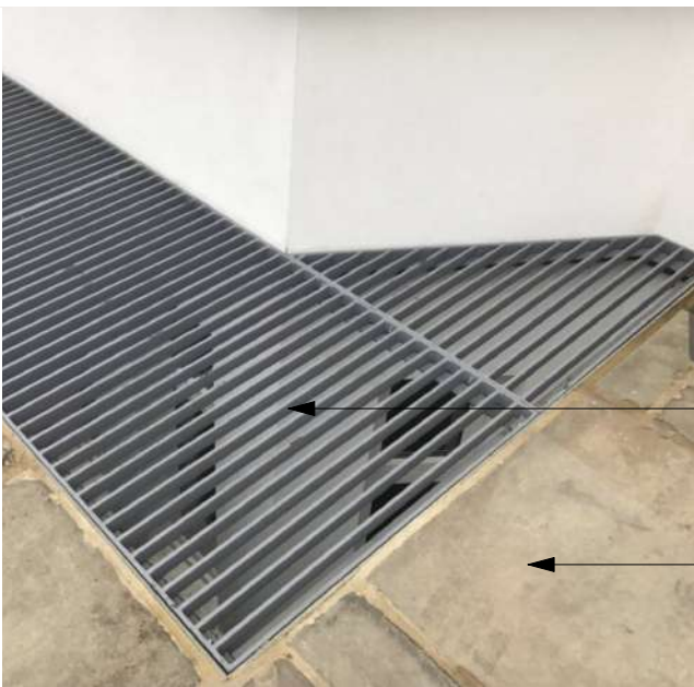
7 - galvanised steel grille to lightwell, flush with paving
