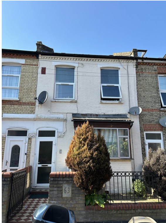
Plate 1. The front elevation of 63 Park Ridings from the footway, showing the forecourt, boundary wall and railings. The bin enclosure is proposed within this forecourt.
