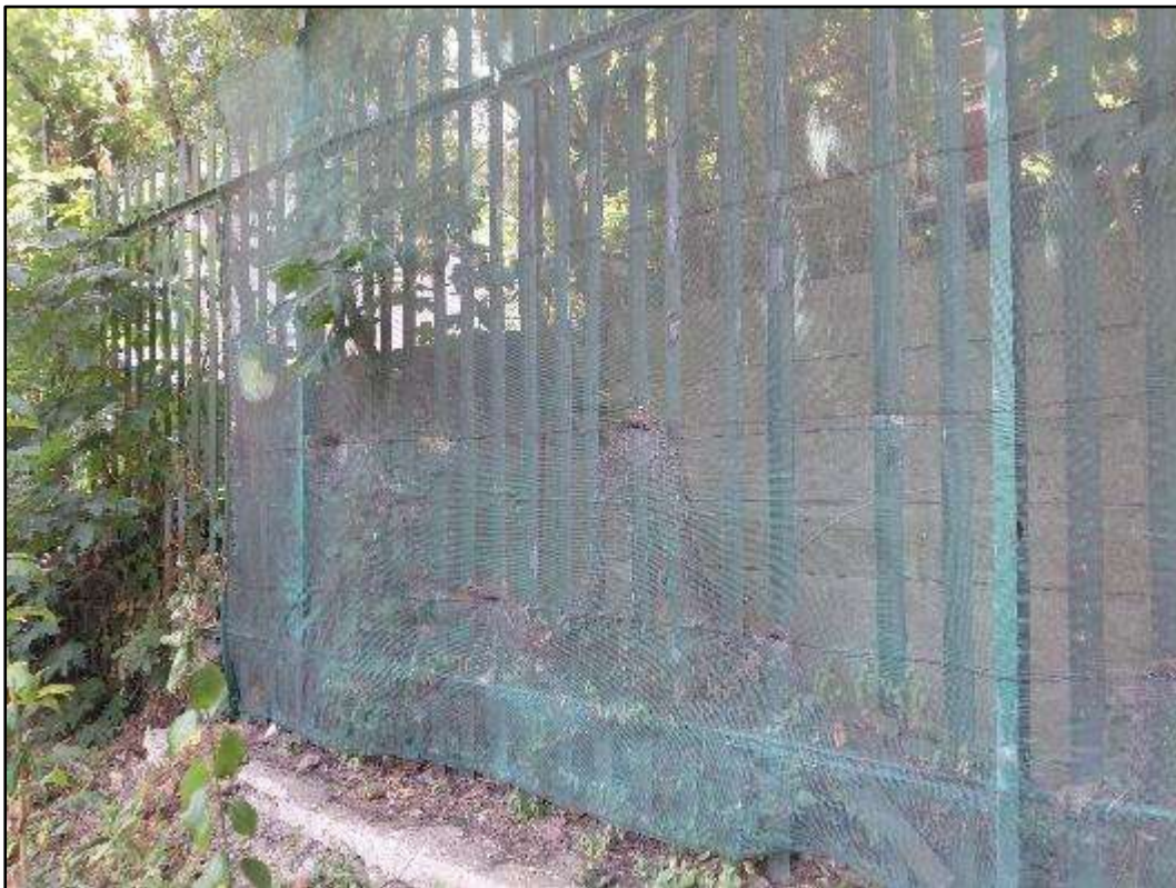
Plate 6: retaining wall within the southwest corner containing the majority of scrub trees G10.
