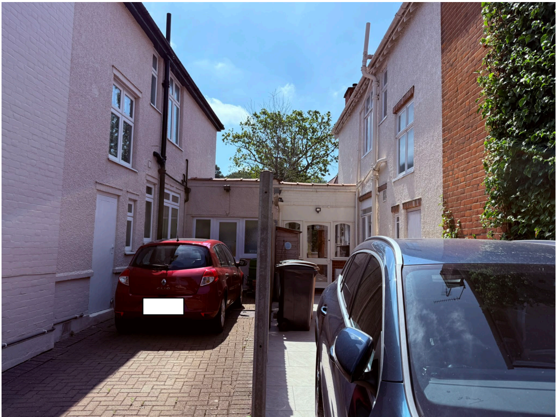
View of the front elevation.
