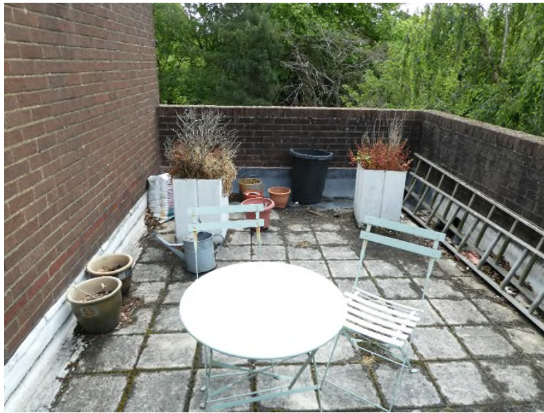
01: Terrace roof looking towards the right hand end.
