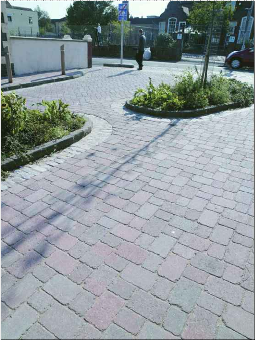
SETTS PERMEABLE PAVING, UPSTAND & LOW LEVEL PLANTING
