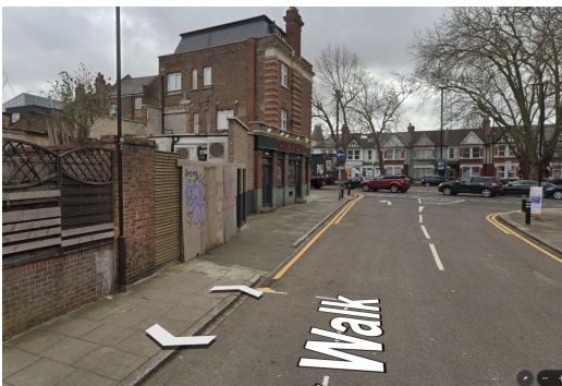
View to unloading zone on Willow Walk
