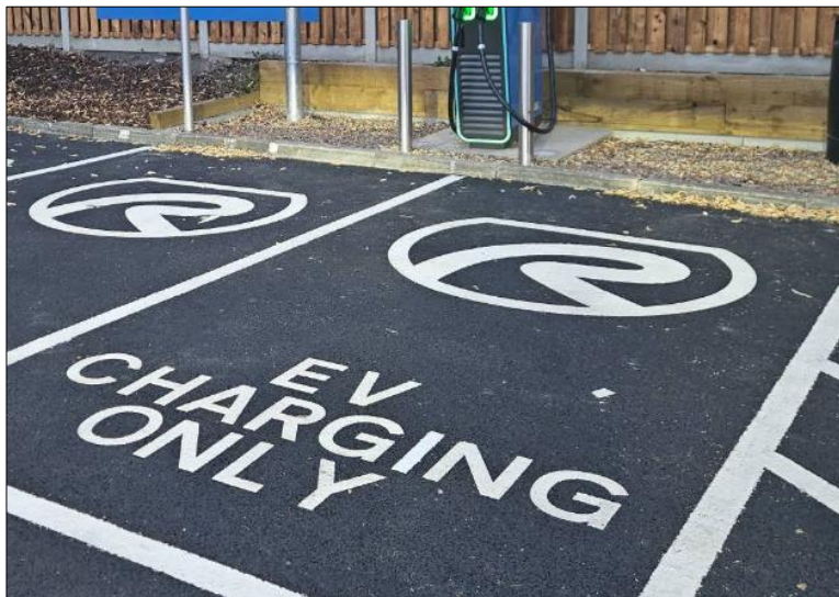
Figure 6A Surface Marking
