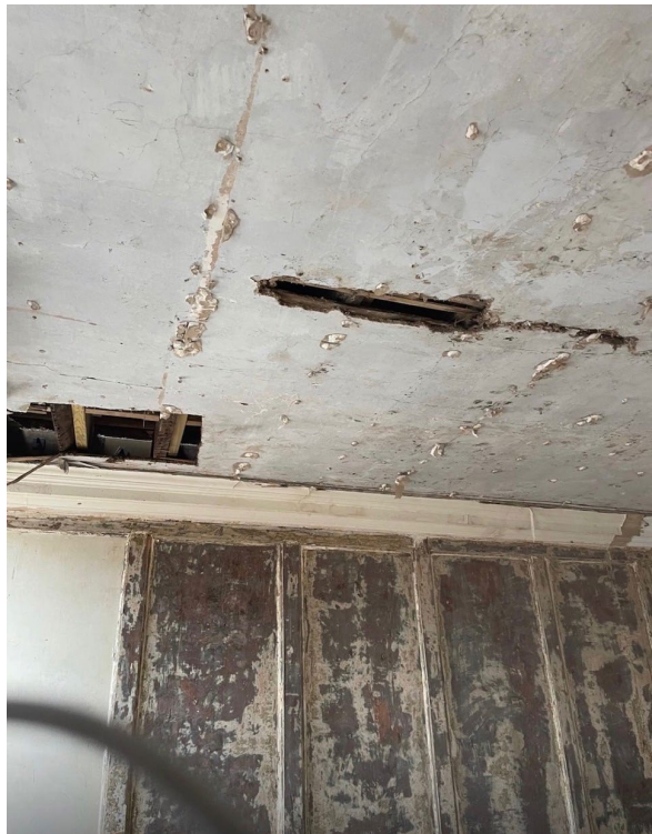
Fig.3 (left): Fractured and displaced laths with extensive dark staining consistent with prolonged water saturation of the ceiling structure. Fig.4 (right): Openings through the ceiling exposing the laths, with perforations from fixings across the plaster surface (Source: Palliass Ltd, July 2026).
