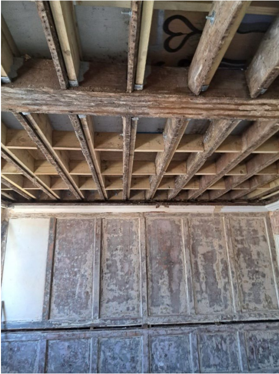
Fig.5 (right): The ceiling as existing with the laths fully removed and the structure cleaned ready for the ceiling reinstatement. Note the modern timbers fitted alongside and between the historic ceiling joists (fitted before the recent works with access from the floor above) using modern joist hangers and threaded bolts to strengthen the structure, evidencing the ceiling required strengthening and stabilisation works.
