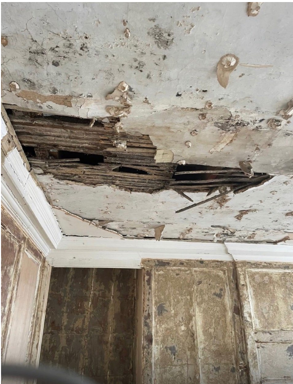
Fig.3 (left): Fractured and displaced laths with extensive dark staining consistent with prolonged water saturation of the ceiling structure. Fig.4 (right): Openings through the ceiling exposing the laths, with perforations from fixings across the plaster surface (Source: Palliass Ltd, July 2026).
