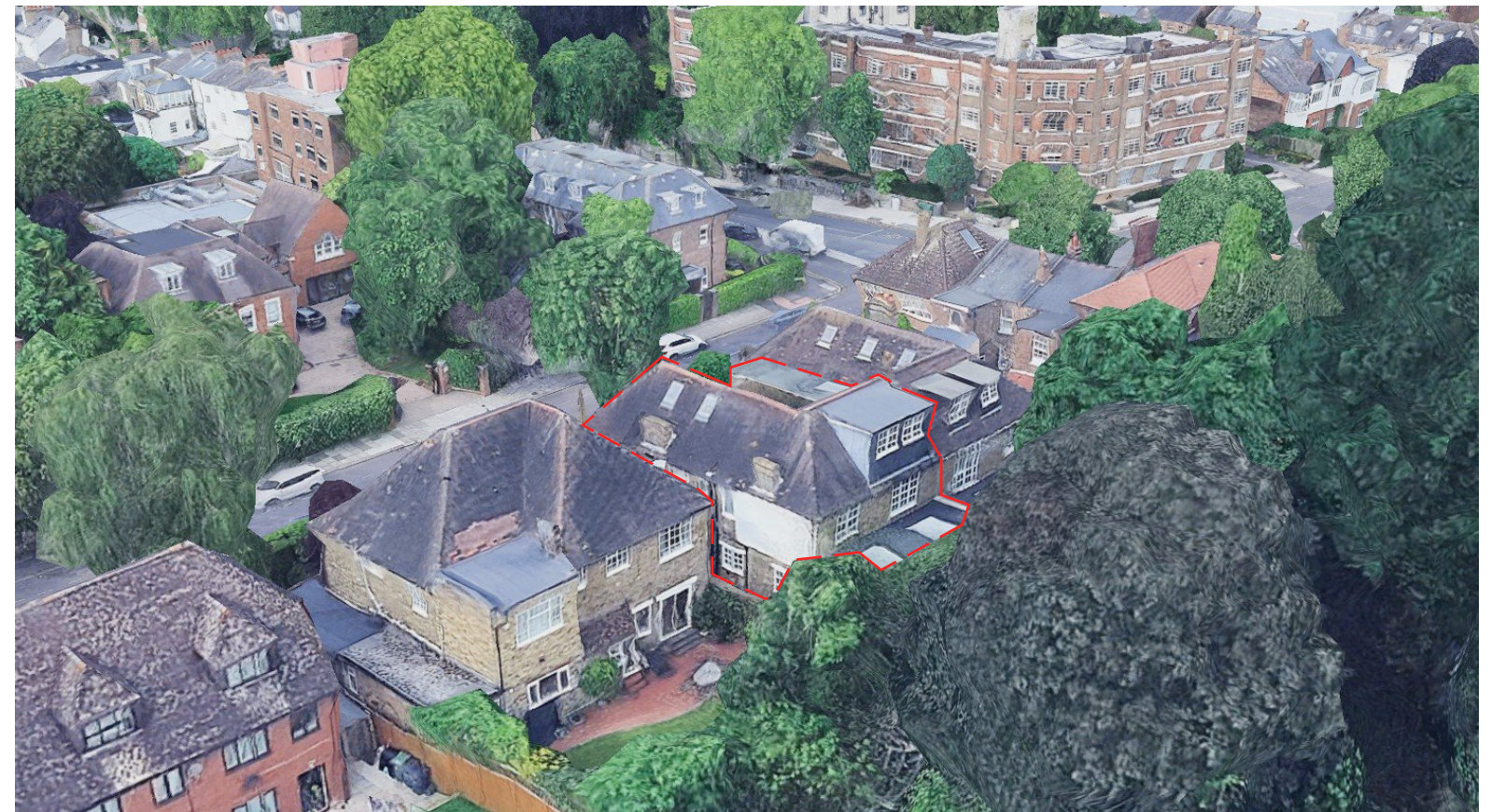
AERIAL PHOTOGRAPHS: MAIN ROAD AND NEIGHBOURING STREETS WITHIN THE HIGHGATE CONSERVATION AREA
