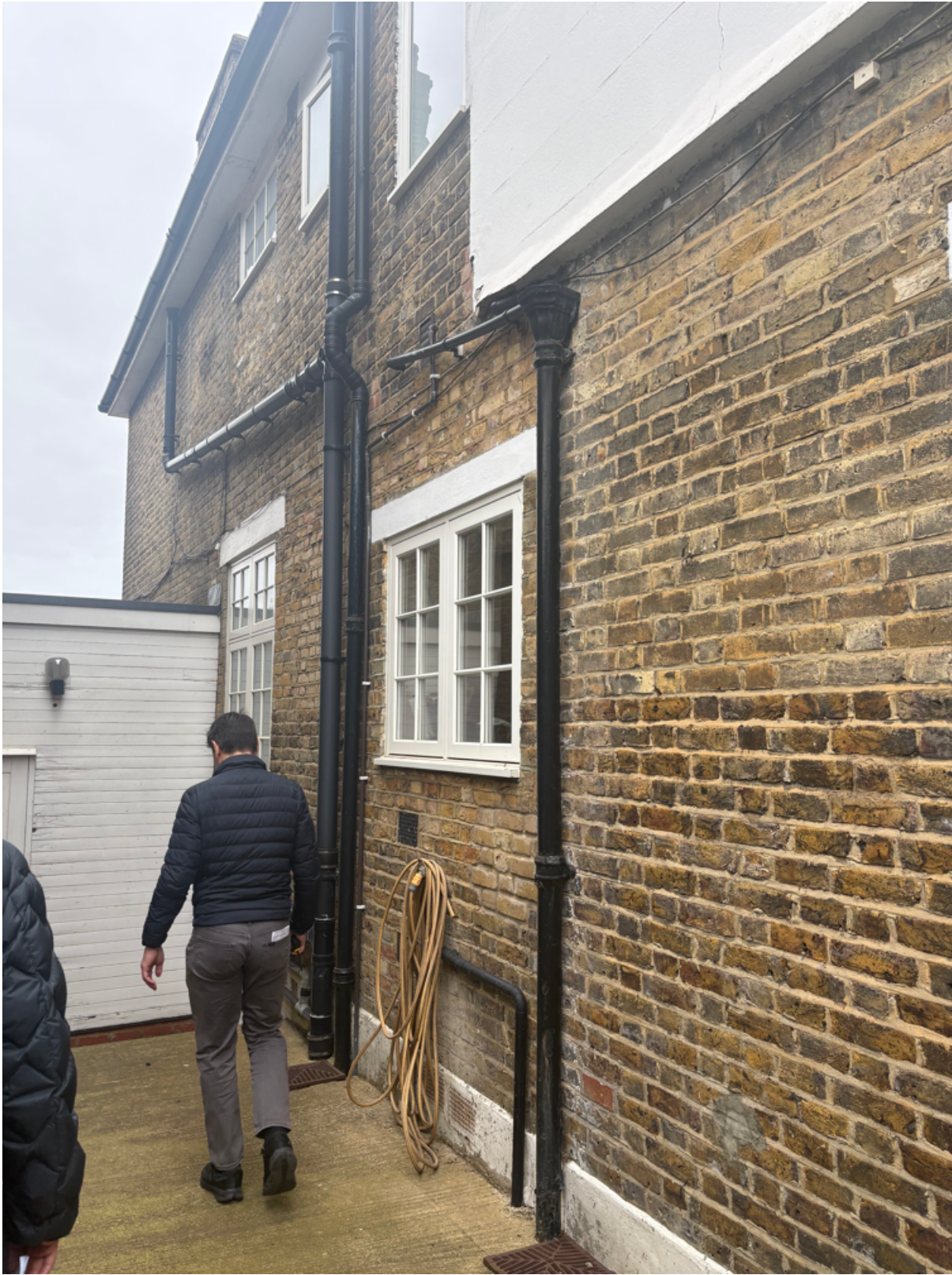
SIDE VIEW: VIEW FROM REAR TO FRONT (FRONT GARAGE)
