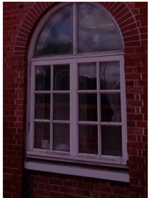
Side Ground Floor Window
