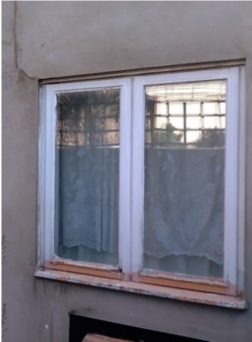
Rear Ground Floor Window
