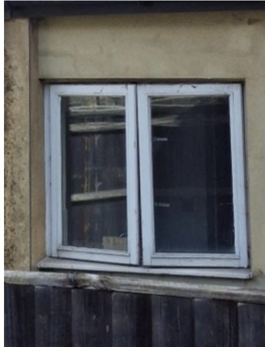
Rear Side Ground Floor Window
