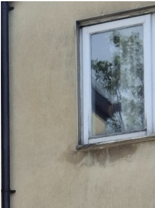
Rear Side First Floor Window
