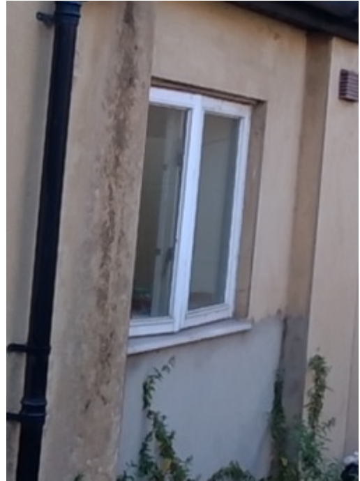
Rear Ground Floor Window
