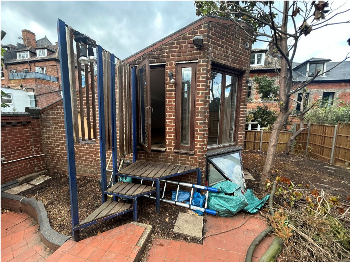
Photograph 04. View of garden building illustrating steps up into the structure and variety of glazing
