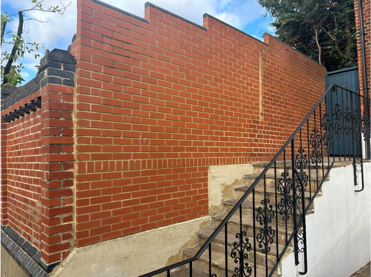
Photograph 10. Existing front driveway steps to number 45 to be removed to be replaced with planting
