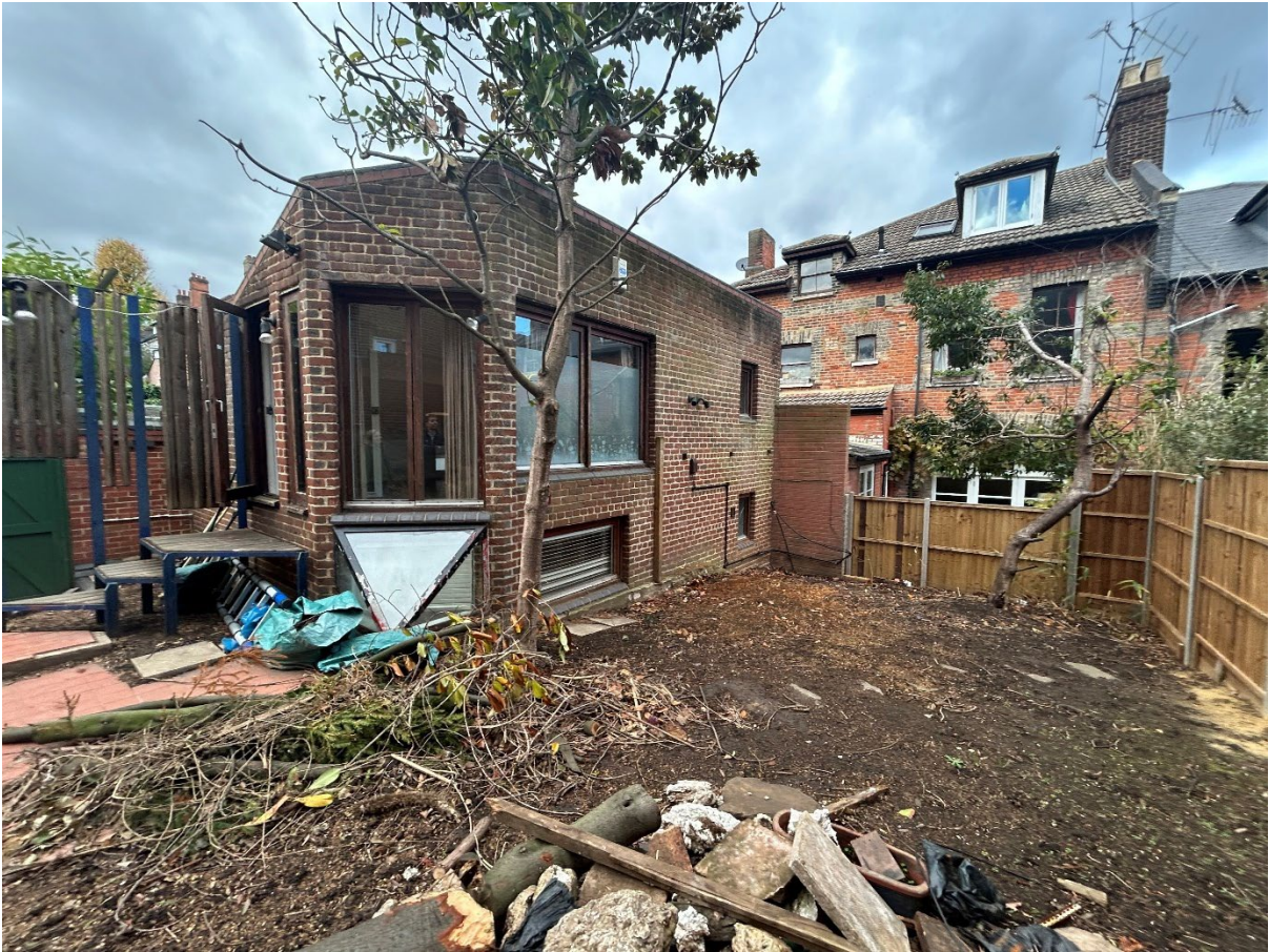
Photograph 05. View of Garden building illustrating diverse range of glazing
