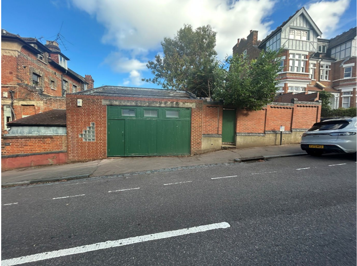
Photograph 02. Illustrating 'poor quality' workshop type appearance to front façade and access opening onto the pavement.
