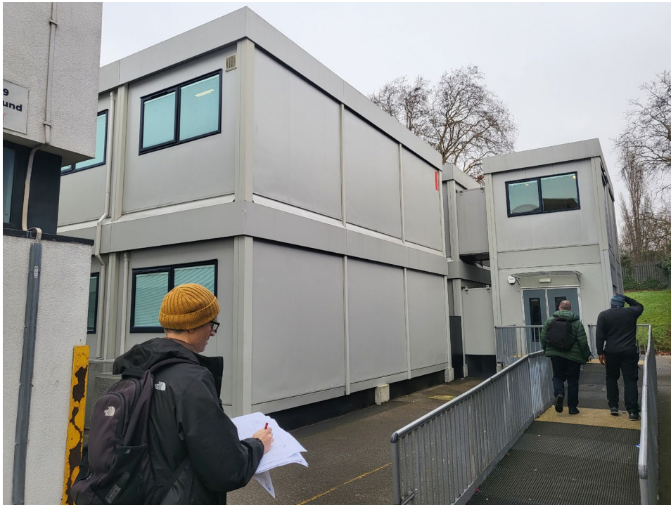
2. Existing view of Temporary General Classroom structure
