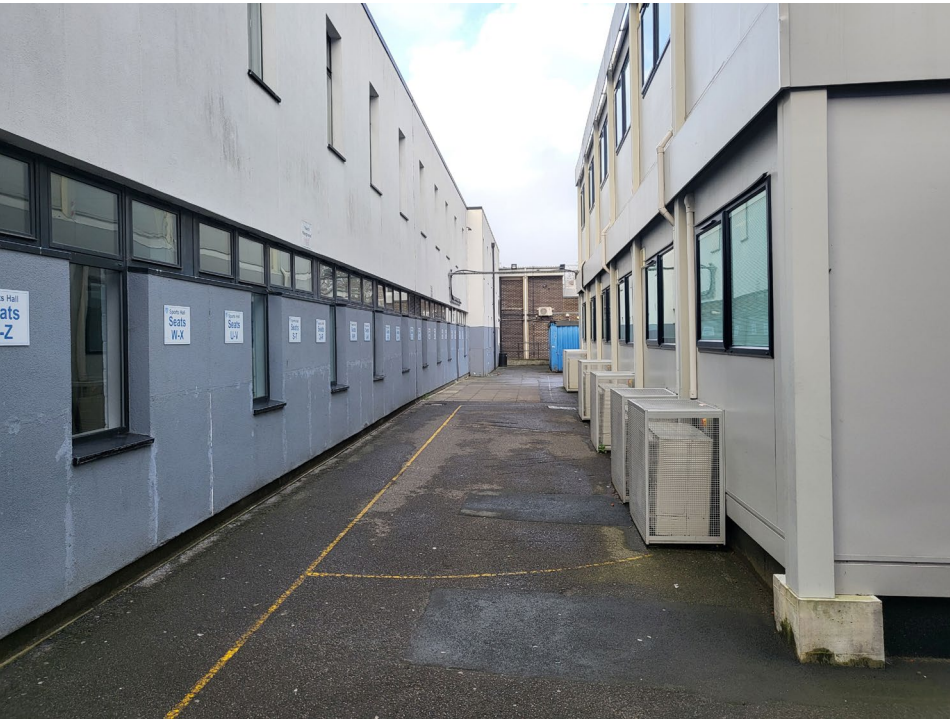
1. Existing view of Temporary General Classroom structure
