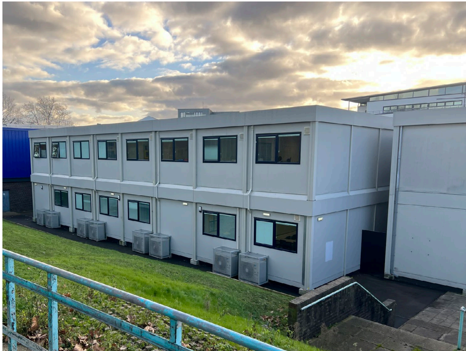
3. Existing view of Temporary General Classroom structure
