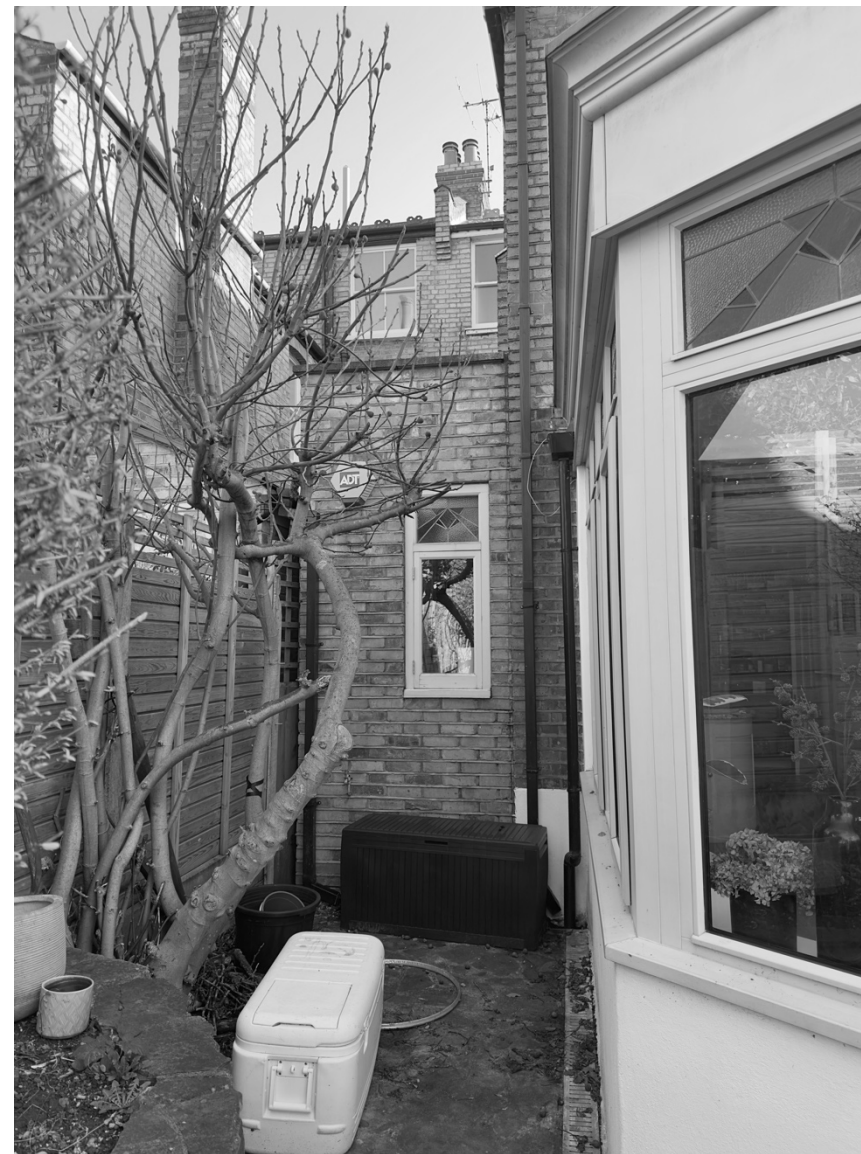
Location of the proposed Air Source Heat Pumps
