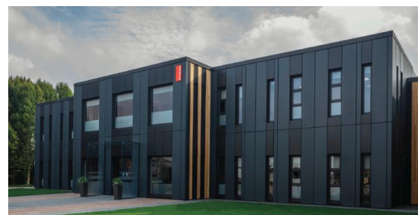
Figure 13 Modular building with external insulation and cladding.
