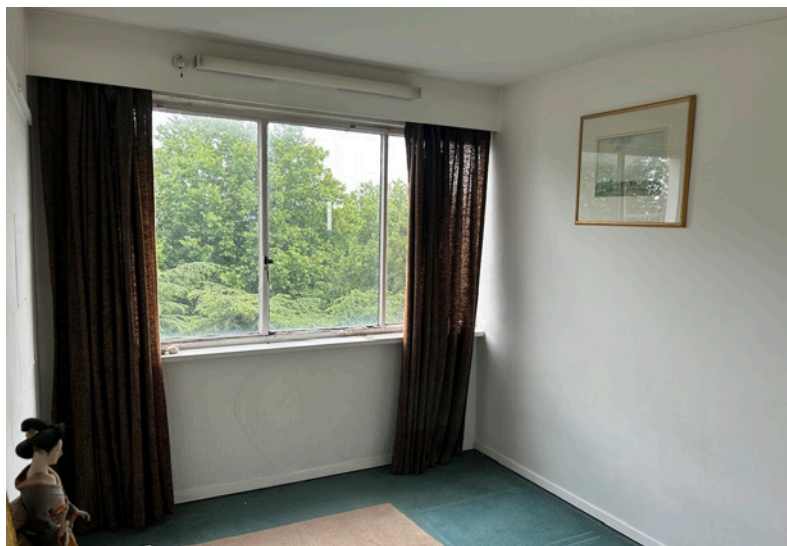
Dressing room - wall to bathroom on right (where new doorway is proposed)
