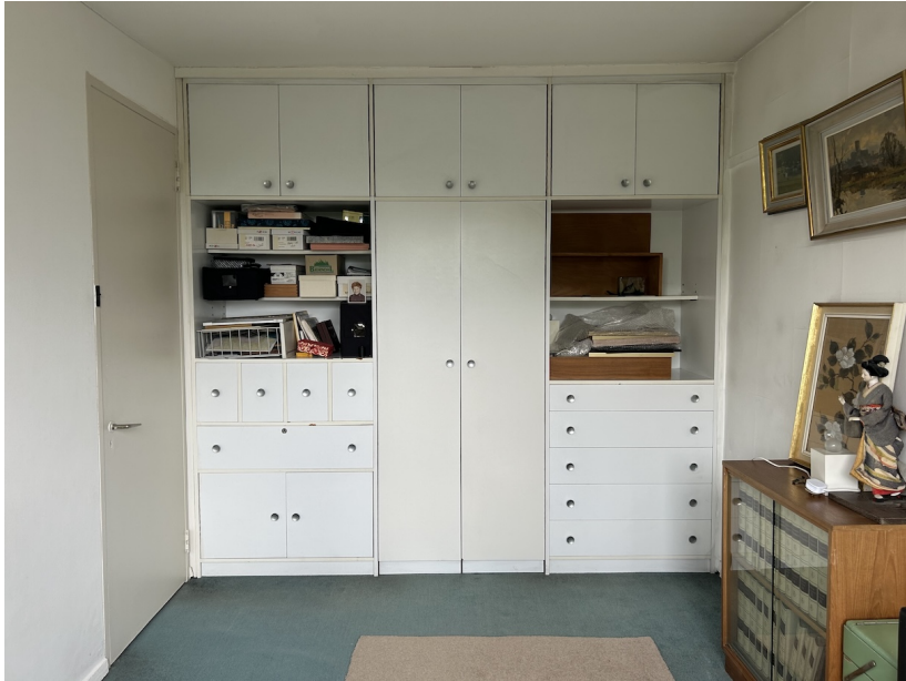
Non-original fitted wardrobes in Dressing Room (proposed to be removed)
