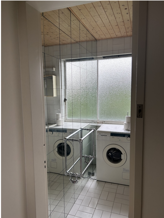
Mirrored wall tiles on left to be removed (along with all non-original bathroom fittings and finishes) Proposed new doorway from Dressing Room would be on the left Original heated towel rail being retained - relocated along this wall
