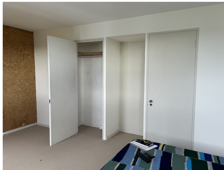
Proposed new open doorway at rear of cupboard on left (door from bedroom retained)
