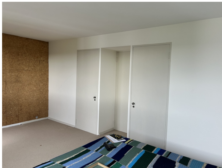
Door to Landing in centre with cupboard doors either side
