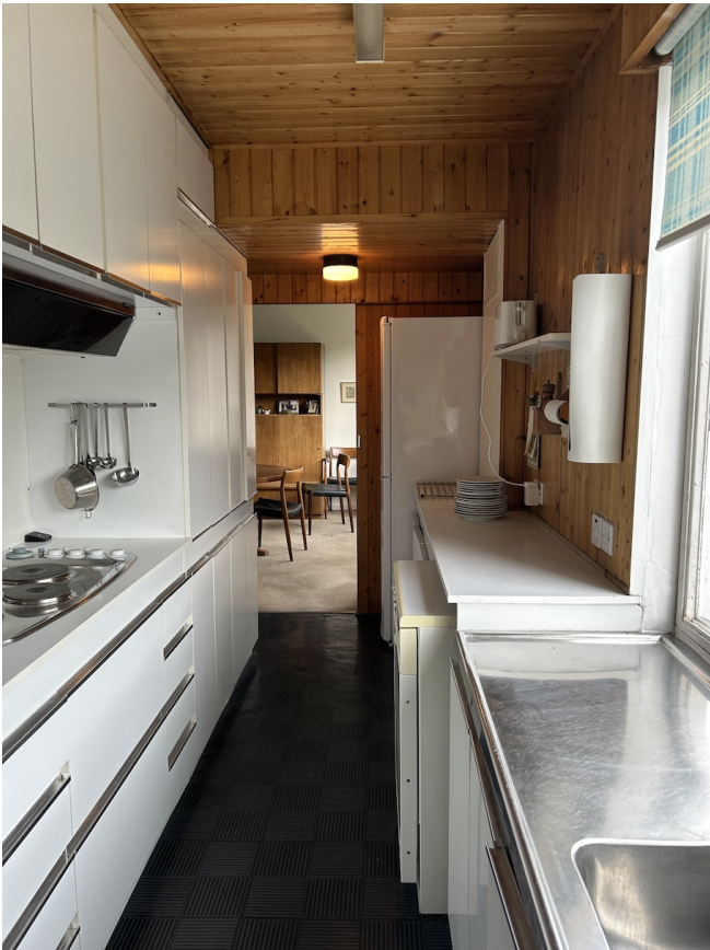
Existing kitchen - view from hallway door. All fittings and finishes proposed to be replaced.
