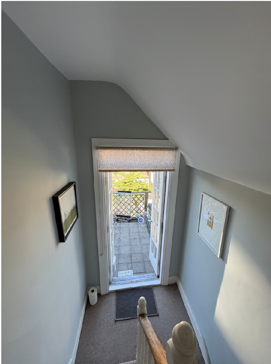
(Existing photo showing access doors and walk-on terrace)
