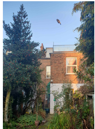
View from rear garden towards house
