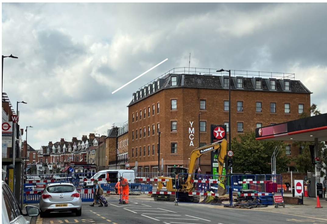
View looking south on Tottenham Lane indicating the potential impact of the increased height and bulk of the proposed building
