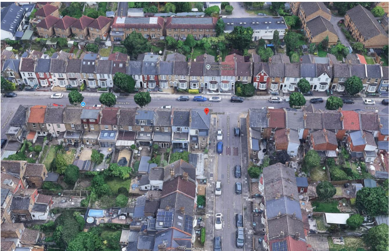
Fig 3. Aerial view of existing site from north (Google).
