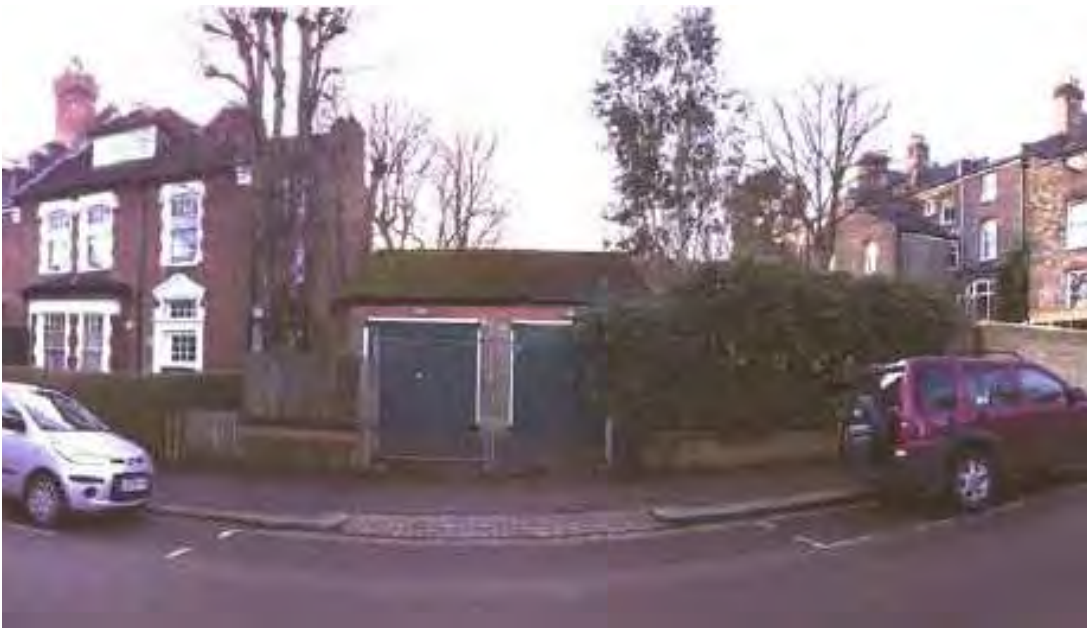
Previous Existing Garages
