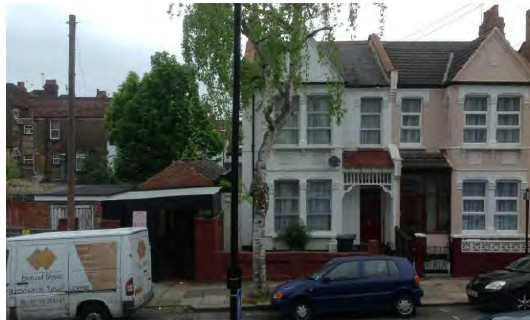
Previous Existing Garages
