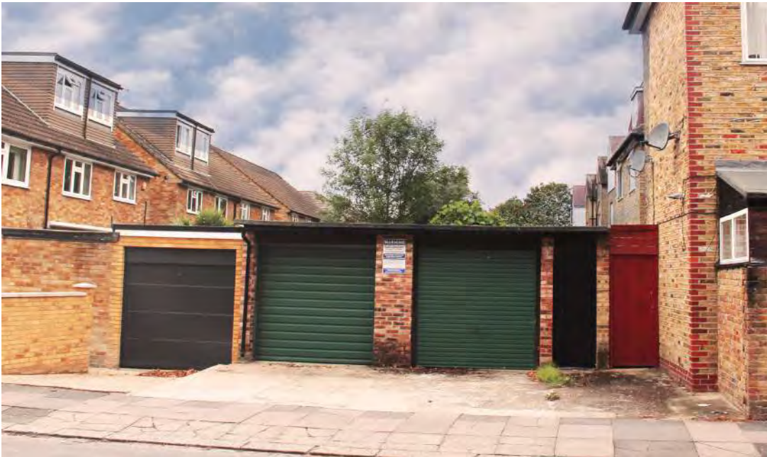
Previous Existing Garages
