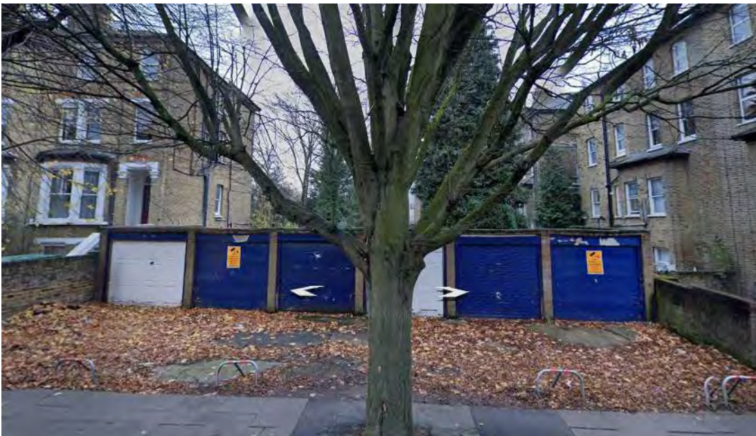
Previous Existing Garages
