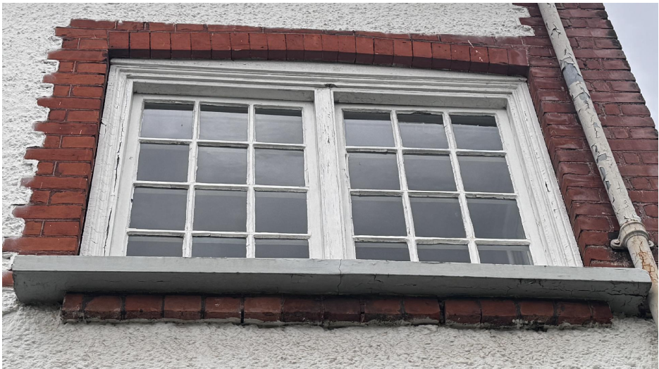
Picture of the existing window
