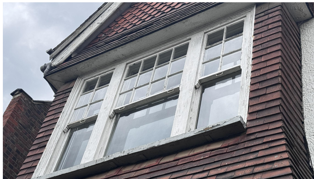
Picture of the existing window
