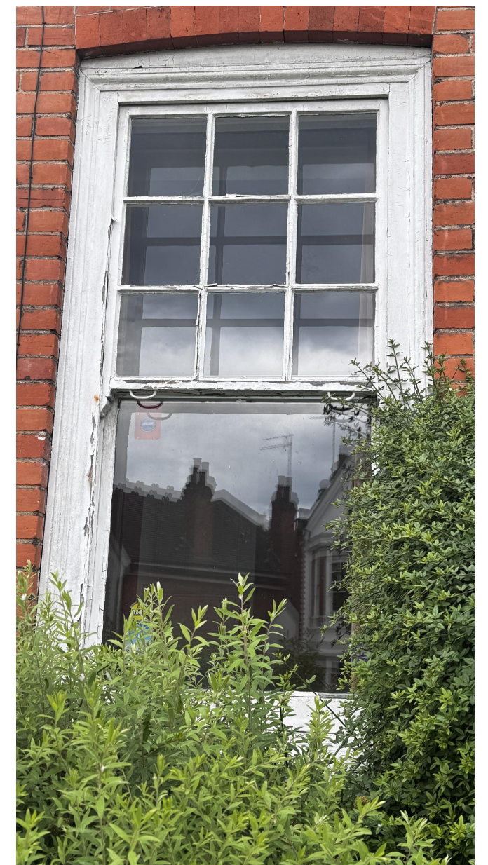
Picture of the existing window
