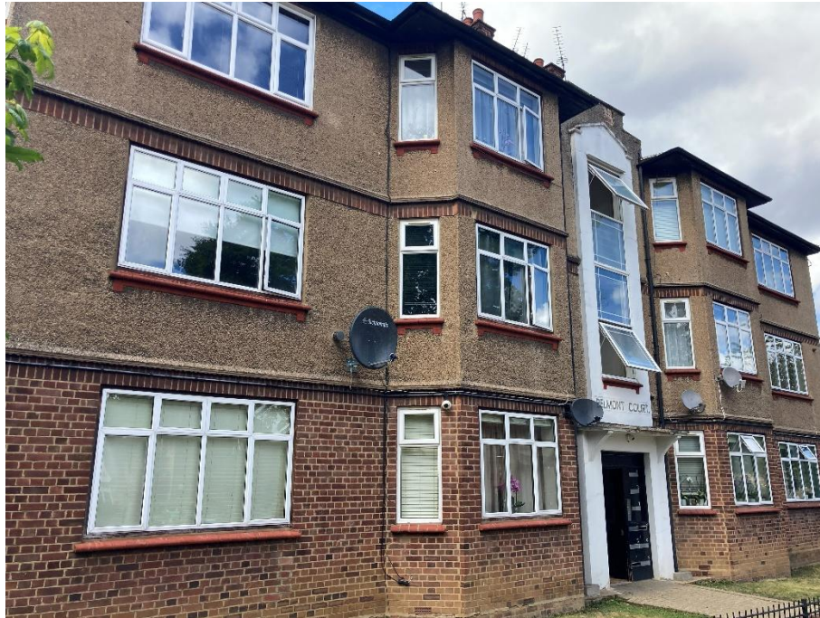
Photo 5 - Southern aspect of the existing building with access to Gordon Rd
