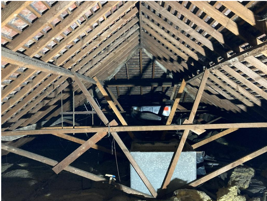
Photo 1 - Roof space of the existing building.
