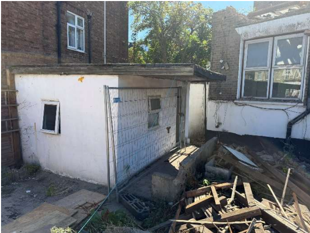
Print 13 View of single storey extension
