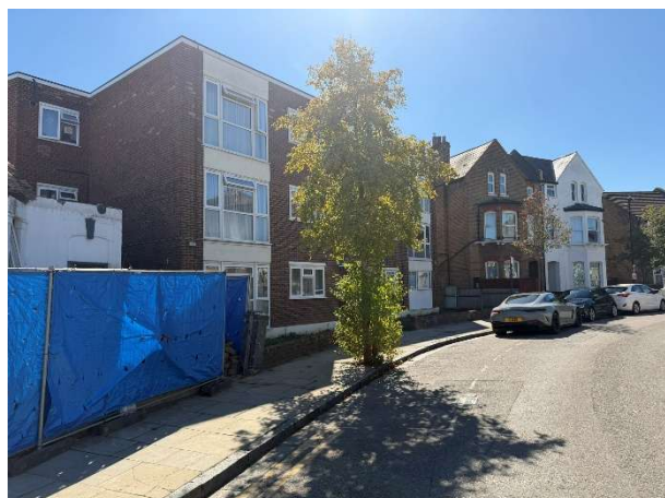
Print 19 View from the front of the site
