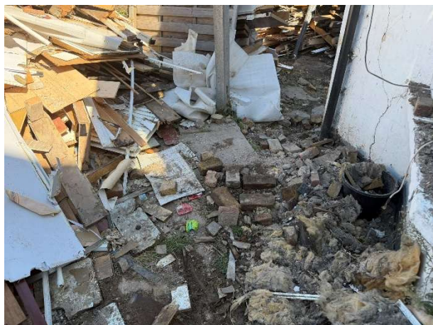
Print 4 View of demolition waste
