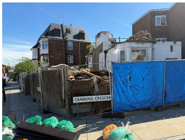
Print 20 View from the front of the site
