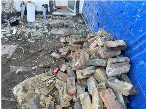
Print 2 View of demolition waste
