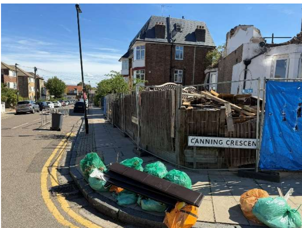
Print 17 View from the front of the site
