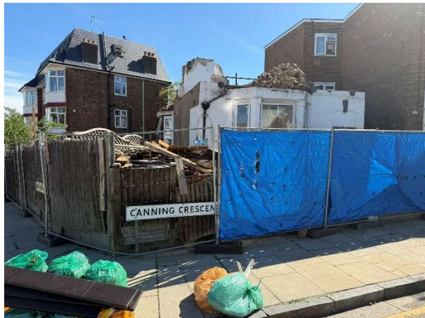
Print 16 View from the front of the site
