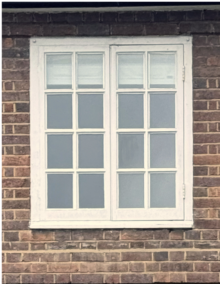
Existing Photograph Existing Window Type 01B
