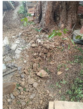
P06 – External – Ground Conditions near the tree
