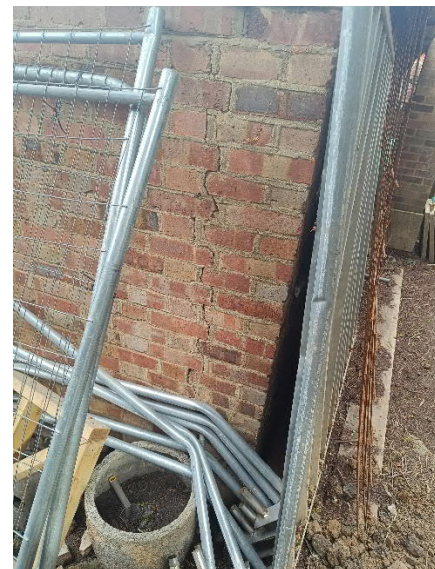
P08 – External – Nearby Structure Opposite to Tree location
