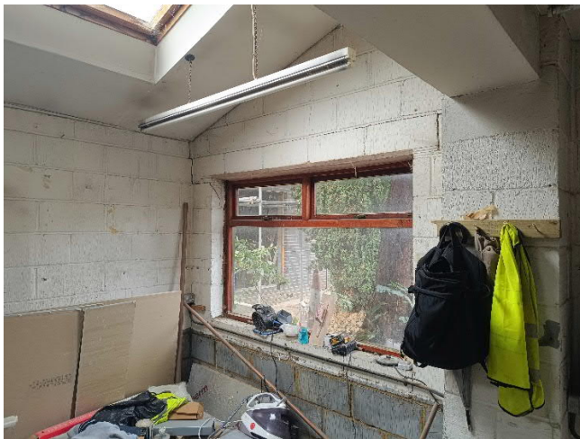
P01 – Internal – Single Storey Building
