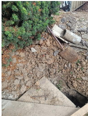
P05 – External – Ground Conditions near the tree
