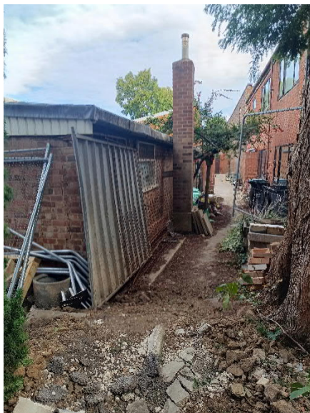
P07 – External – Nearby Structure Opposite to Tree location
