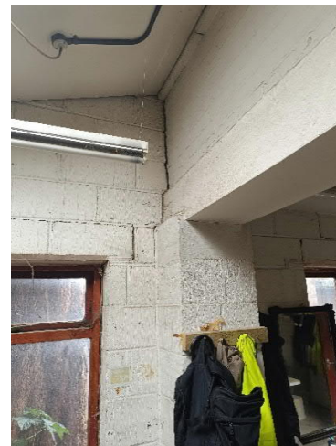
P02 – Internal – Single Storey Building
